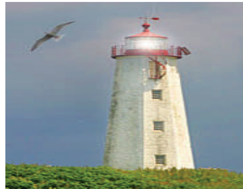
Faulkner's Island lighthouse
